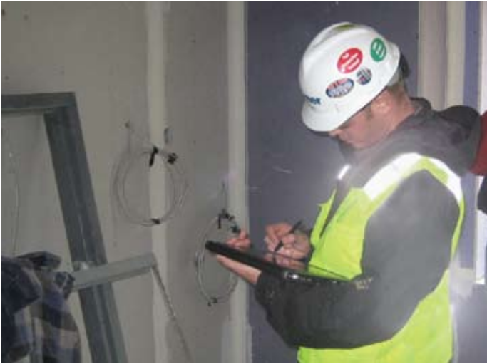
Turner personnel using Vela Systems on 10 Rittenhouse Square
