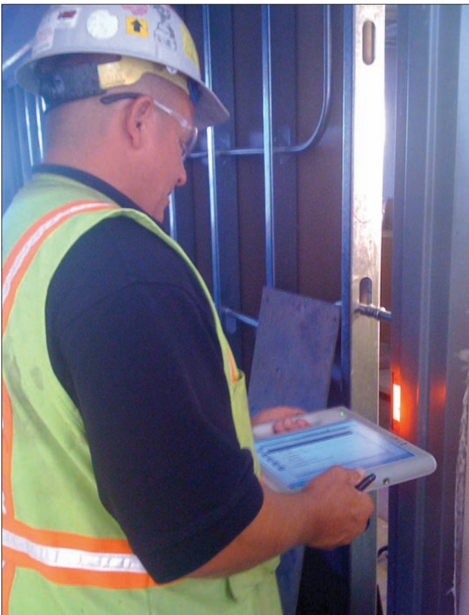
Darrin Sterlinski: DFH Foreman for the UCSC Porter B project scans a Frame Assembly
